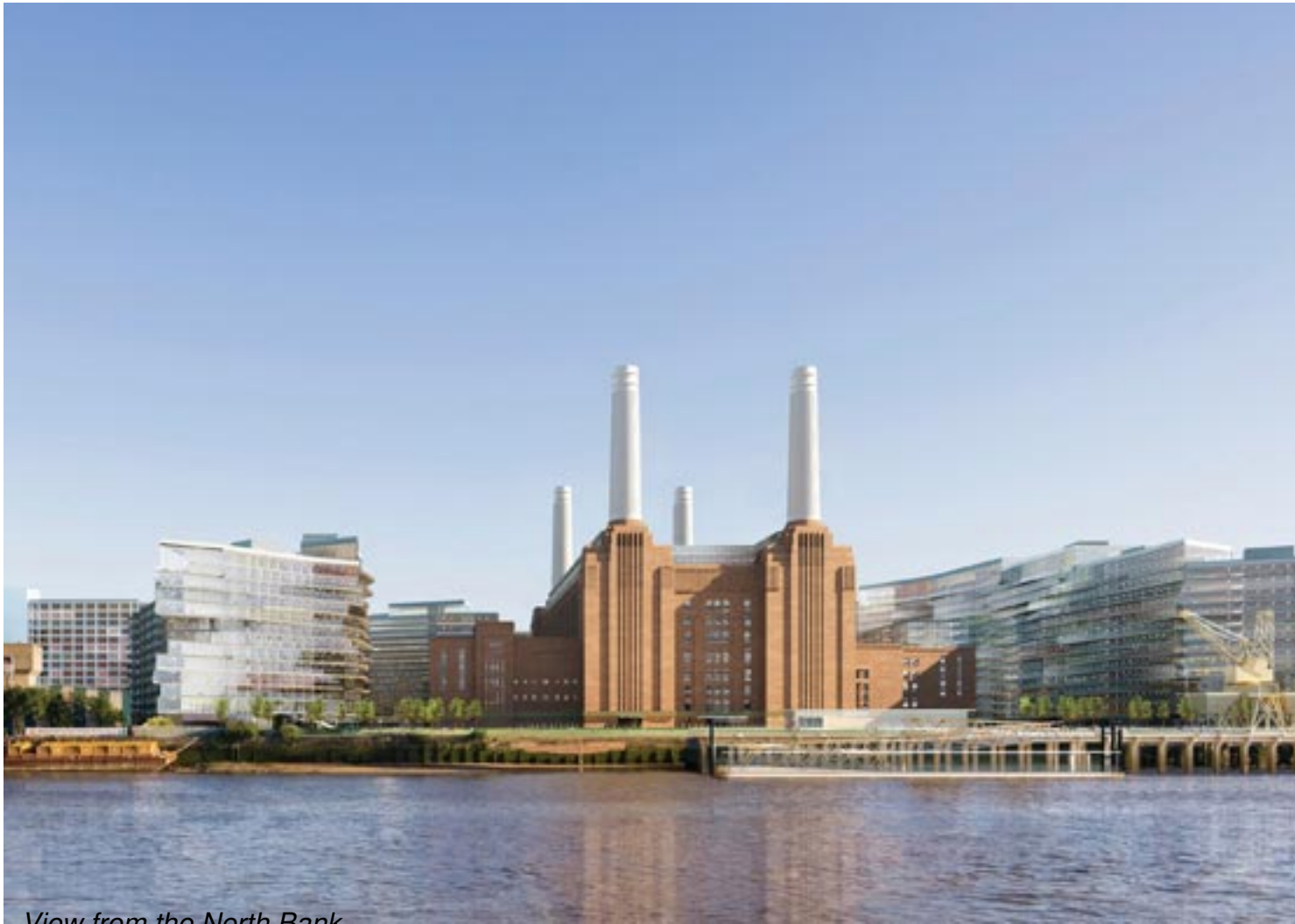
View from the North Bank
