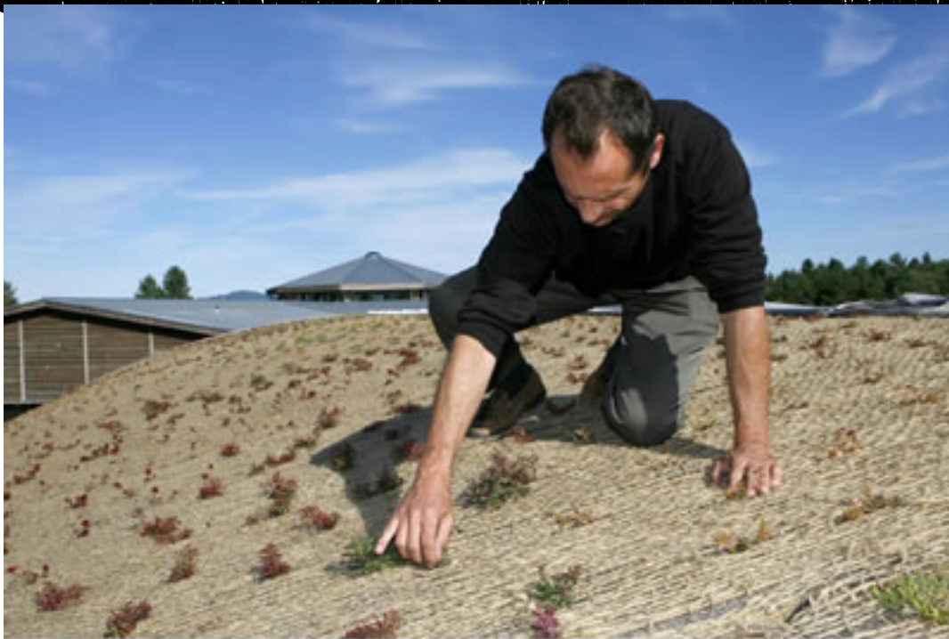
Planting seedlings on the Green Roof of the Bio Building
