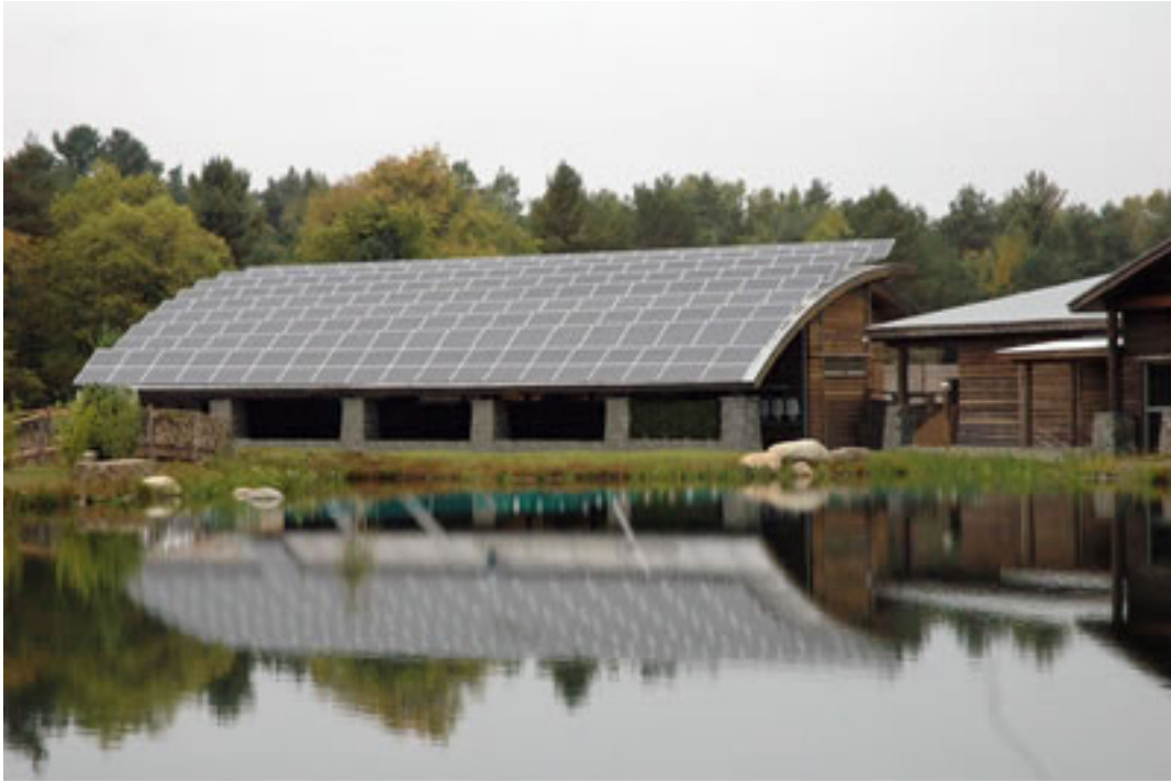
Solar panels cover the roof of Bio Building
