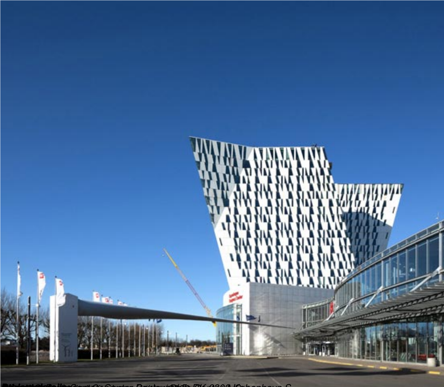
3XN's Bella Sky in Copenhagen, DK nears completion A photograph of the Bella Sky building in Copenhagen, Denmark, featuring a distinctive white and black geometric facade and a glass-walled lower section. A construction crane is visible in the background.
