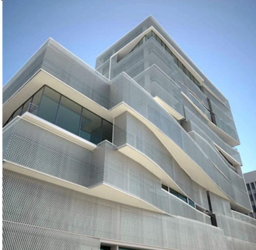
Exterior view of the Taipei Tower facade, highlighting the perforated metal screens and the stepped design.
