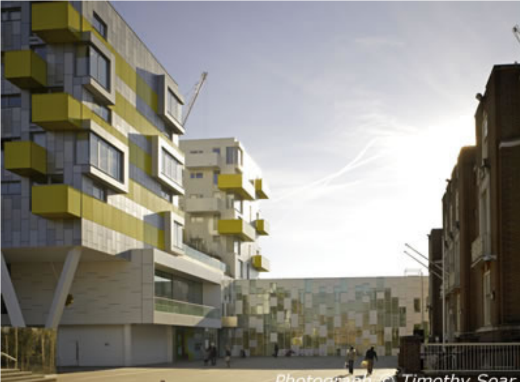
Photograph © Timothy Soar. The building is supported by a concrete structure.
