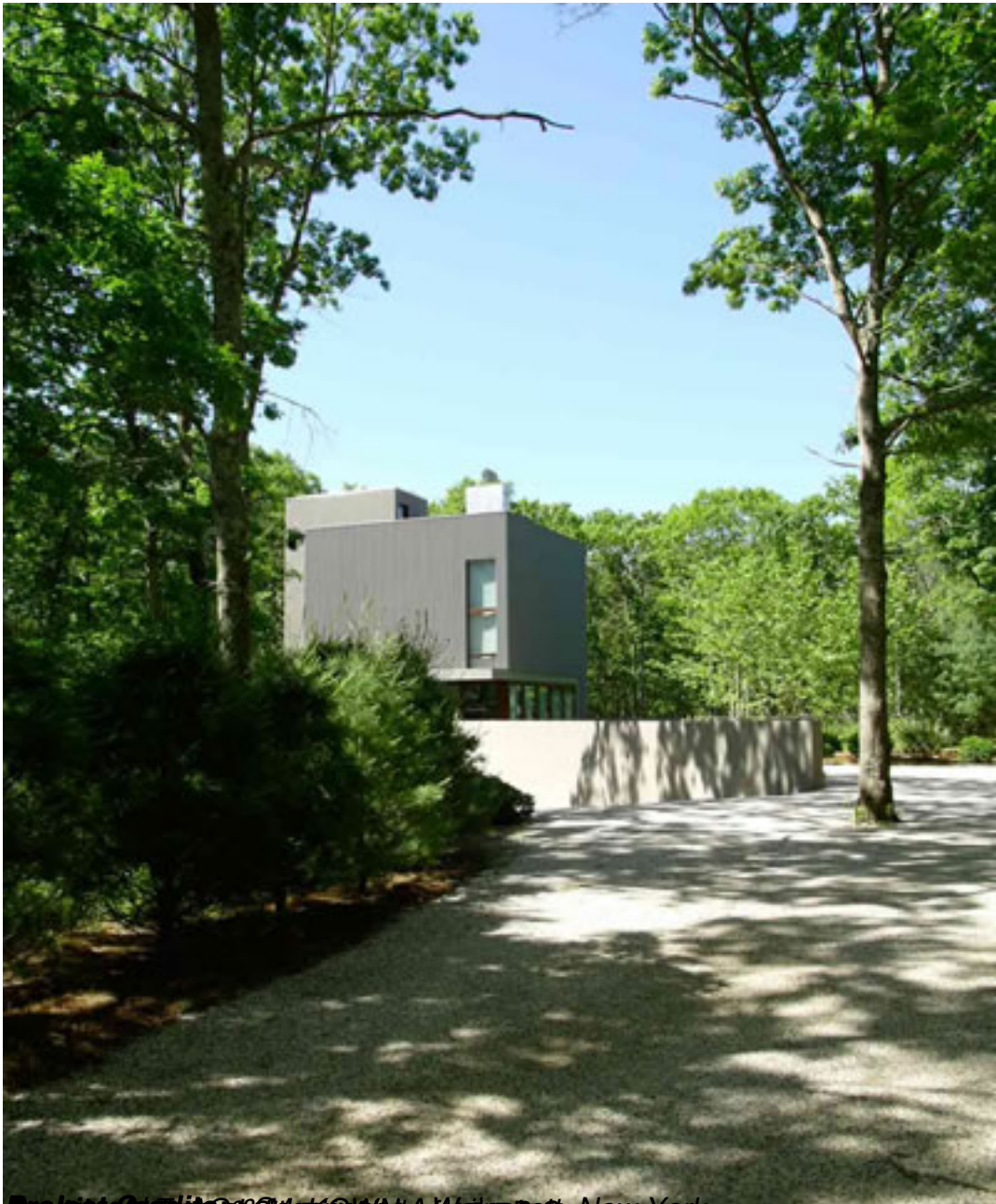
Project: House at Sagaponac in Wainscott, New York. Photographed by William Armstrong Design.
