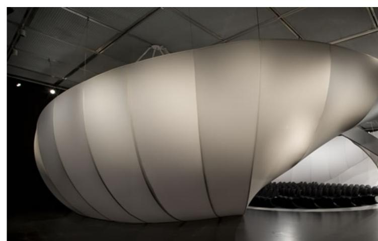
The ribbon itself consists of a translucent fabric membrane articulated by an internal steel structure suspended from the ceiling. The surface of the fabric shell undulates in a constant but changing rhythm as it is stretched over the internal structure.
