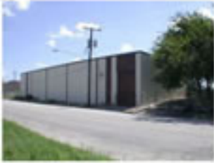
Original existing warehouse.
