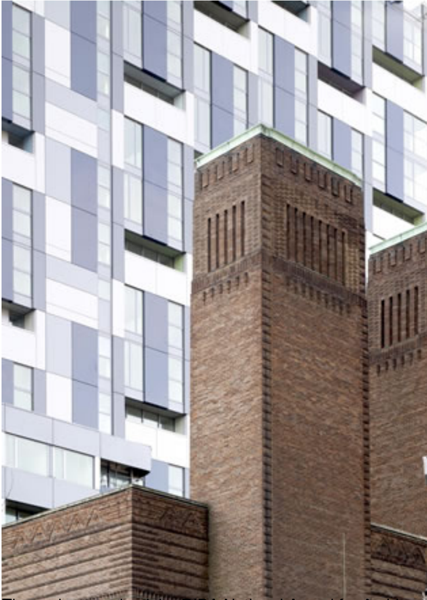
The project received the RIBA National Award for Architecture in 2007
