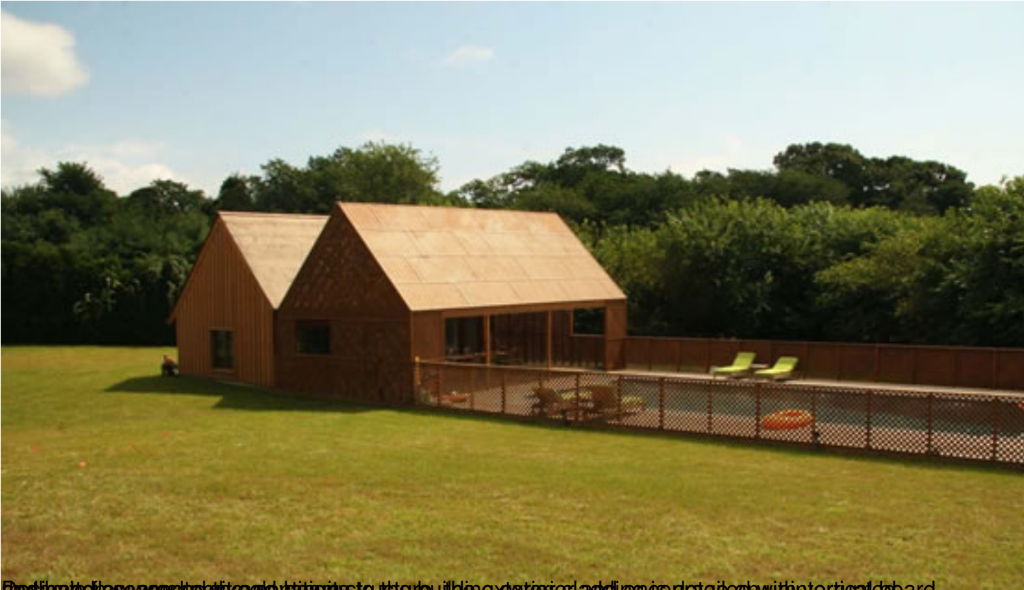
By Sigurd Lewné, the architect of the building, the exterior cladding is designed with vertical board
