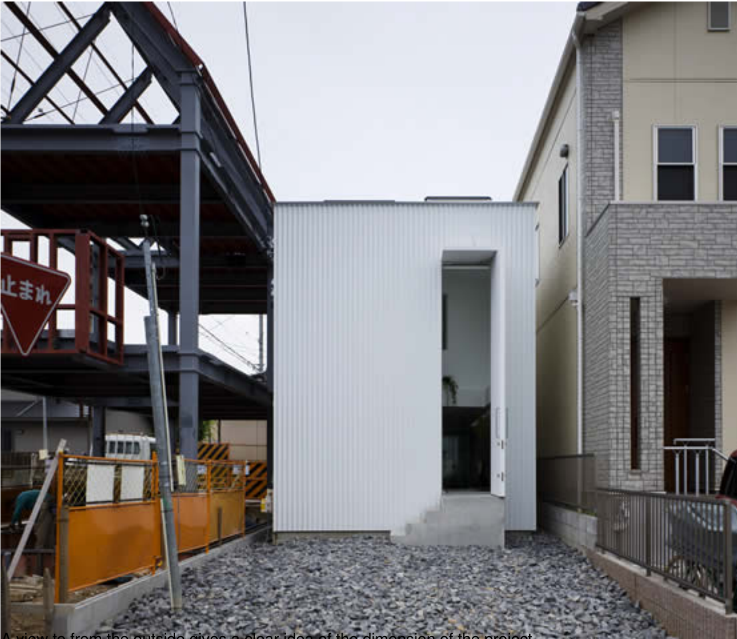
A view to from the outside gives a clear idea of the dimension of the project.
